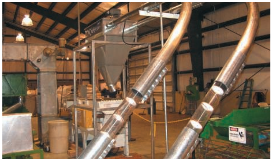
Close-up of Inspection Tube shows tea moving.
